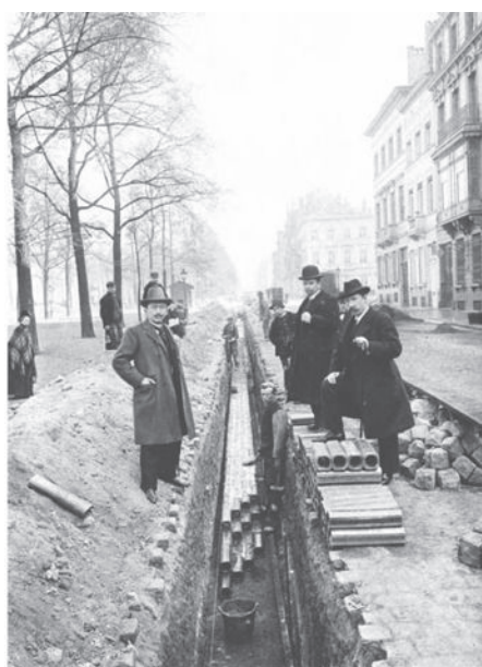
Fig. 6: Installing underground cable in Brussels Ca 1900
