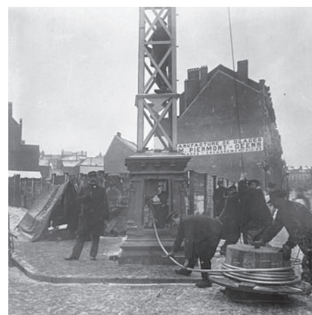
Fig. 7B: Terminating the underground cable
